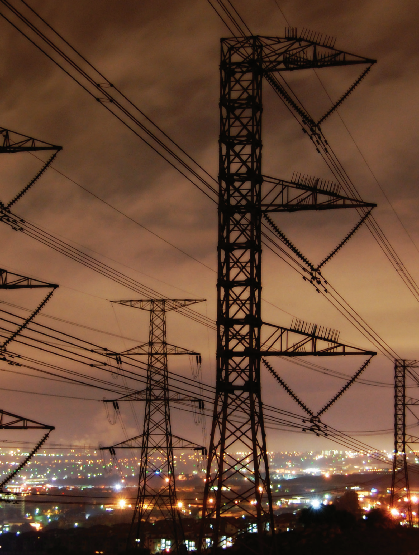
Powerlines in South Africa
